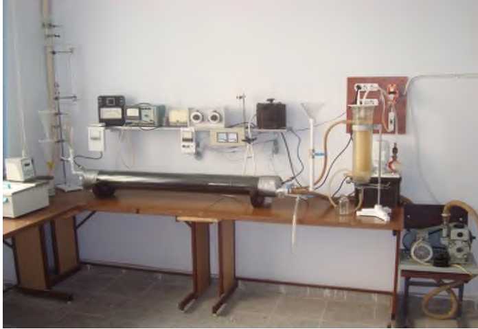
Fig. 24. General view of the laboratory installation of the storage system: solar heat exchanger - helioreactor
