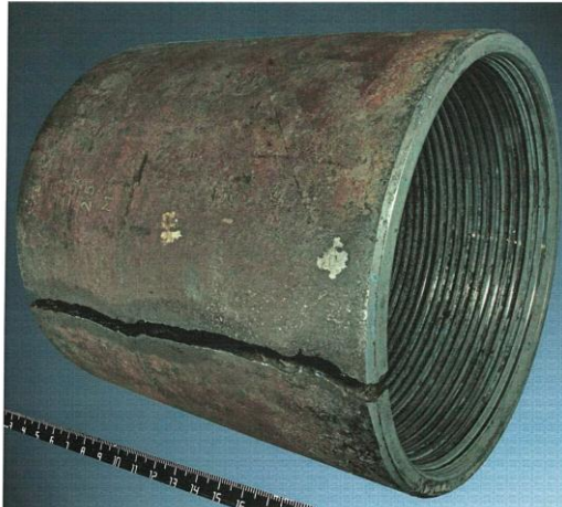
Picture 5. Dispersing of coupling of protective pipe \text{Ø}168 \times 8,9\text{mm} with whole lengthwise crack
